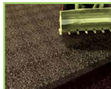
Preparation of the underlying layer
